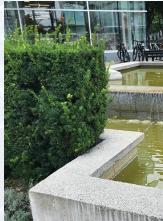
Figure 3. Decorative water feature (did not pass inspection).
