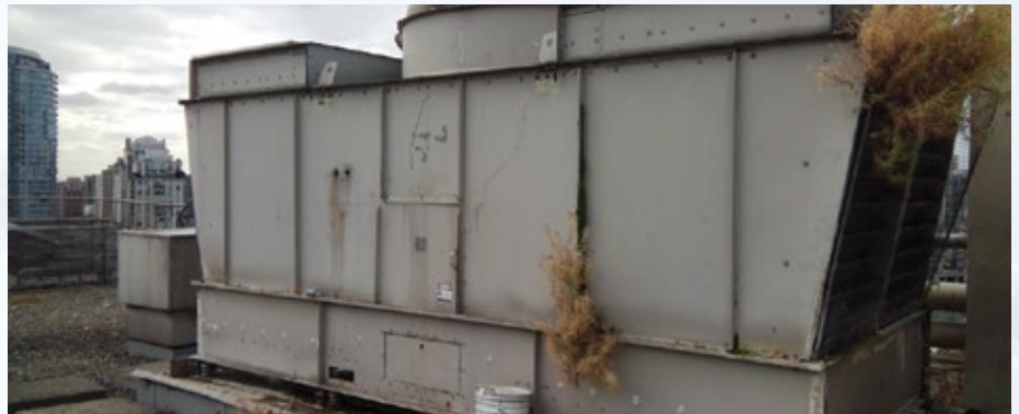
Figure 4. Cooling tower (did not pass inspection).
